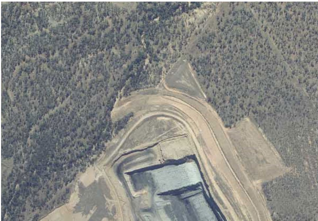
Figure 34. Construction of the Burton Mine void (northern extent) indicated in 2003 imagery, with intact riparian vegetation on the Isaac River immediately north of the pit.
