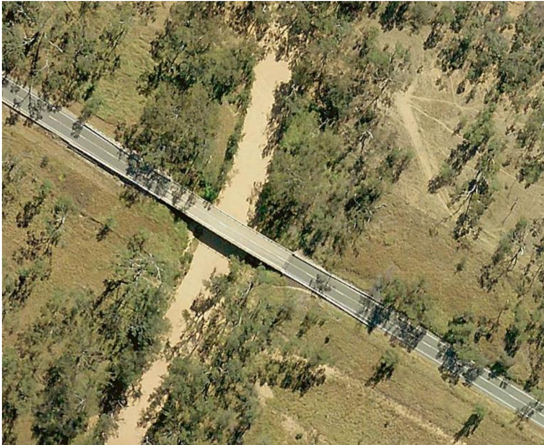
Plate 16: Current Suttor Developmental Road crossing of the Isaac River (source: Queensland Globe)
