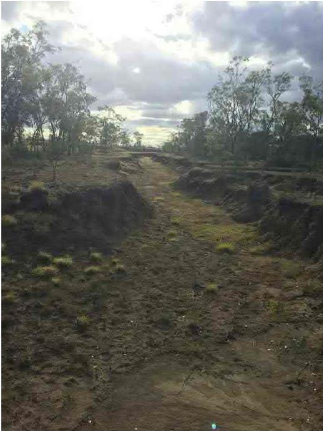
Figure 3.25 Gully erosion to Ti-Tree Creek in upper reaches
