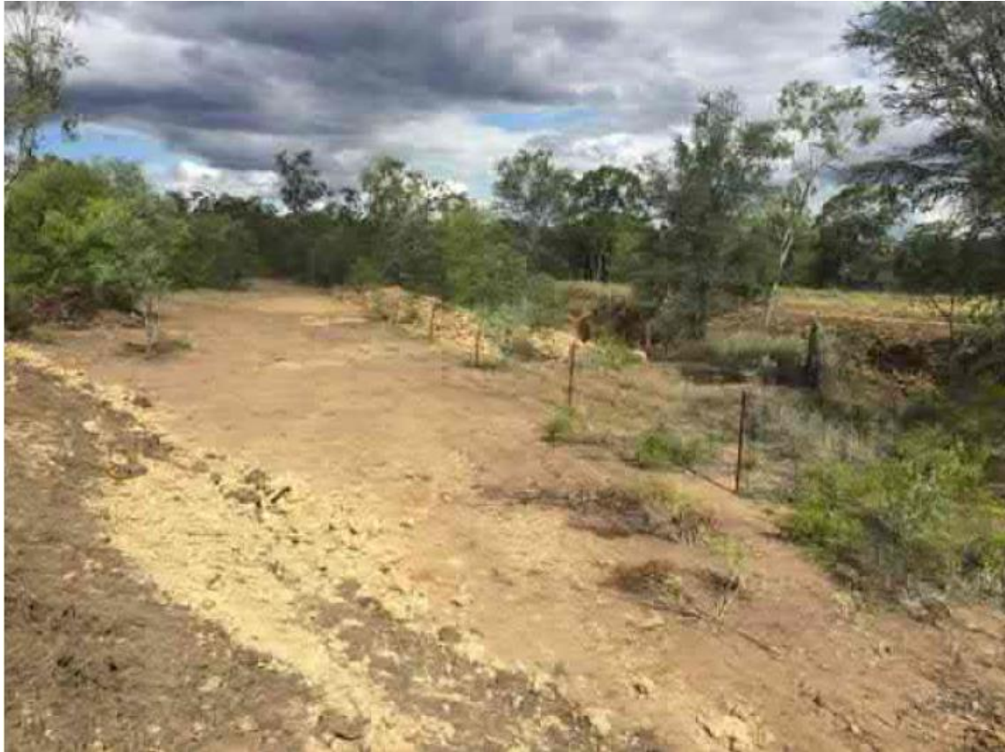
Figure 3.23 Construction of bund to re-direct overland flow away from gully
