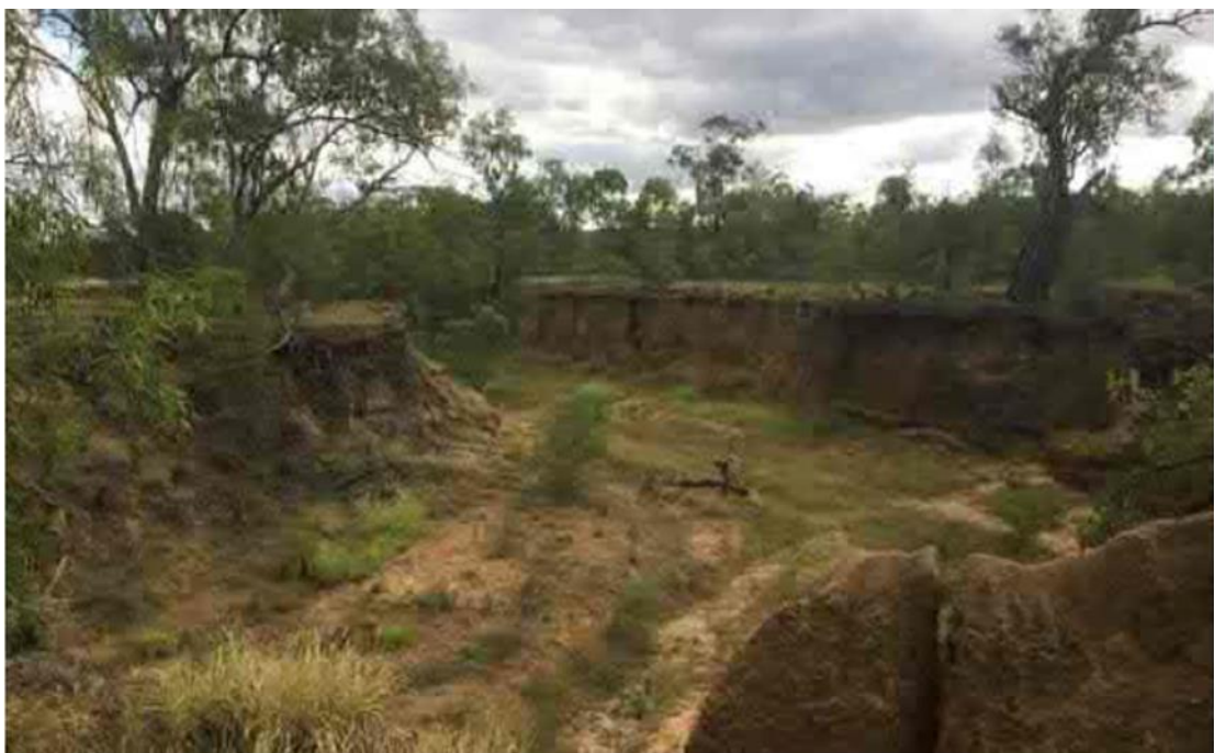
Figure 3.24 Gully erosion to un-named tributary upstream of confluence with Isaac River
