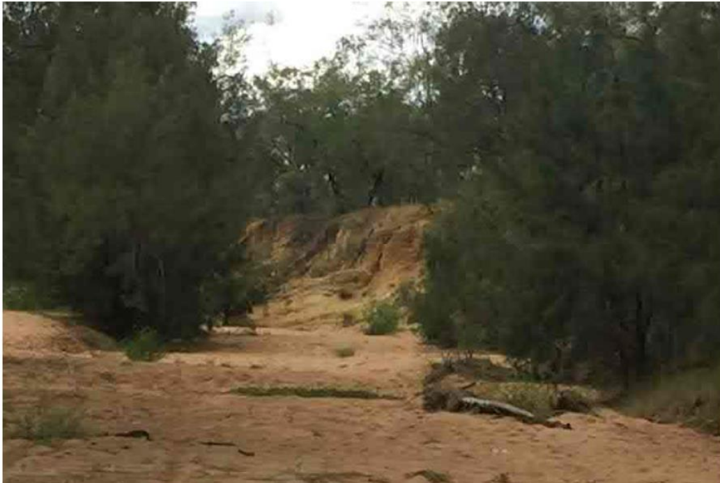
Figure 3.19 Bank erosion evident on outer banks of the Isaac River
