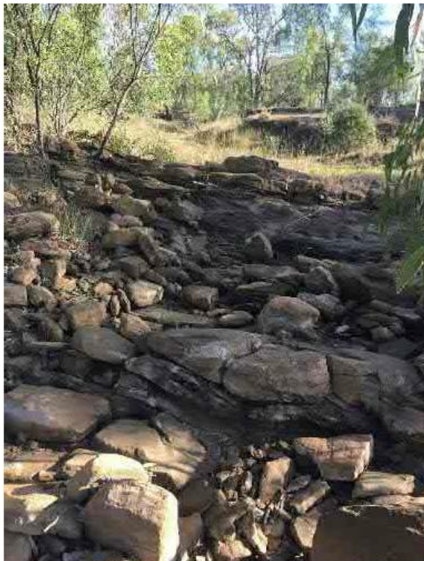
Figure 3.27 Improvement to stability of Ti-Tree Creek – typical for lower sections
