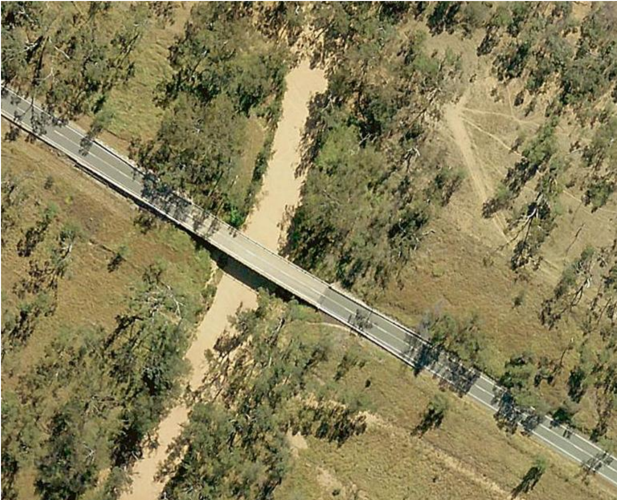
Figure 3-23 Current Suttor Developmental Road Crossing of the Isaac River
