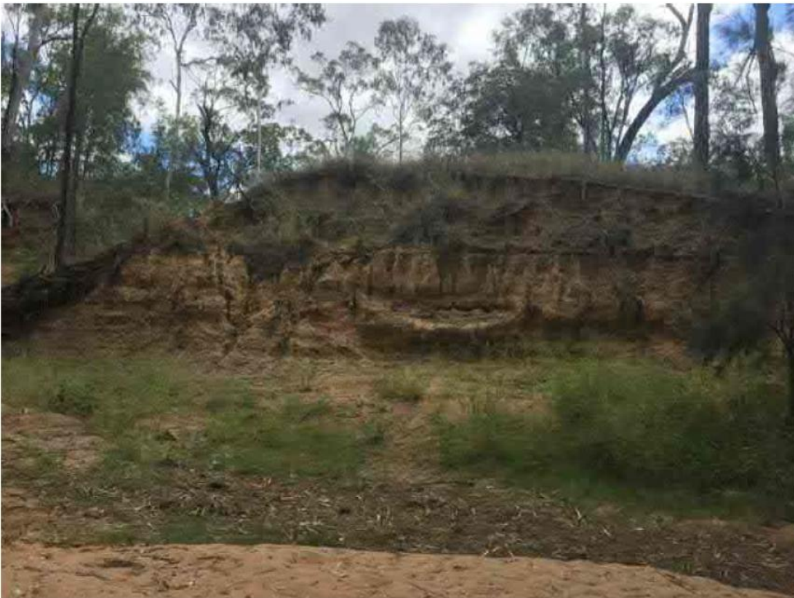
Figure 4-13 Evidence of Bank Erosion, Slumping, Gully Erosion and Aggradation of Sediments on the Isaac River
