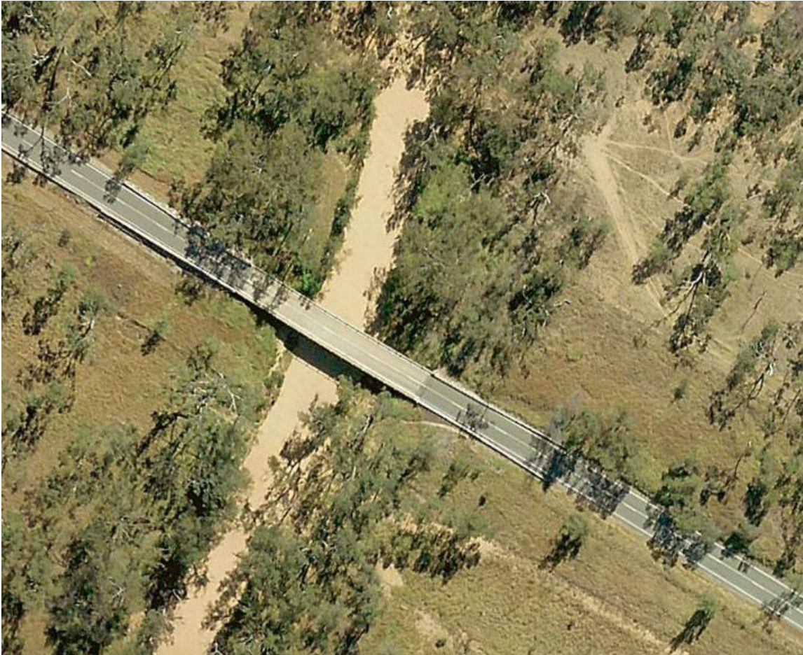
Figure 6-12 Current Suttor Developmental Road Crossing of the Isaac River
